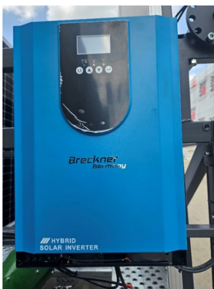
Fig.6. Invertor solar Off-grid 5kW
